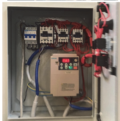
Fig. 10. General view of the convective walnut dryer's control unit
