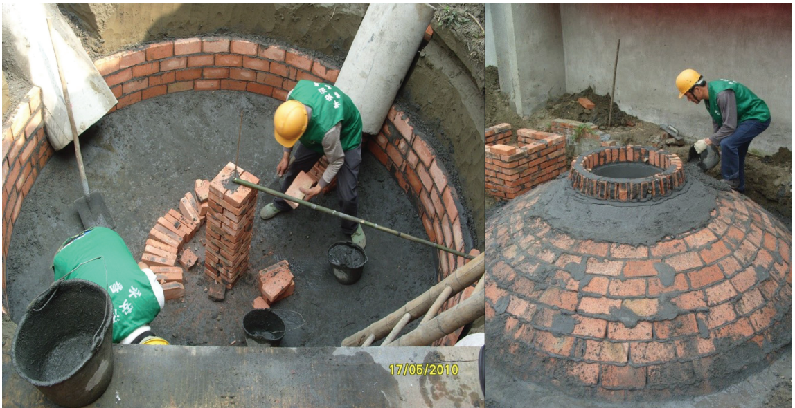
Fig. 4. Biogas plant construction
