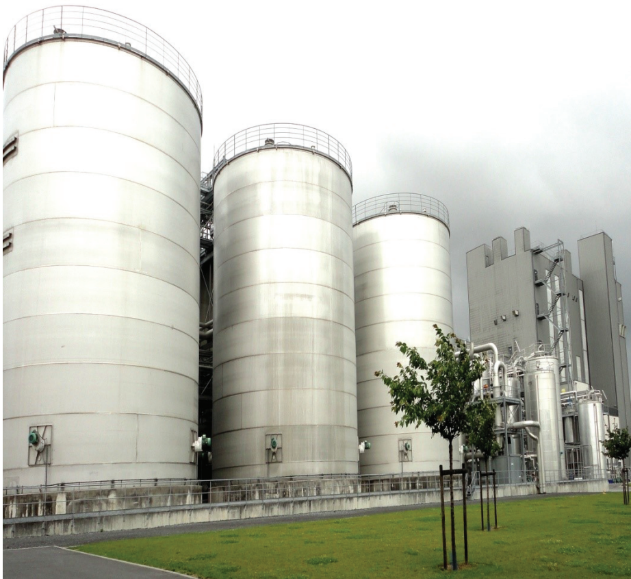
Fig. 1. Cristanol Plant, Basmarkt, France Sugar beets are processed into sugar and bioethanol. Vinasse is exposed to anaerobic fermentation
