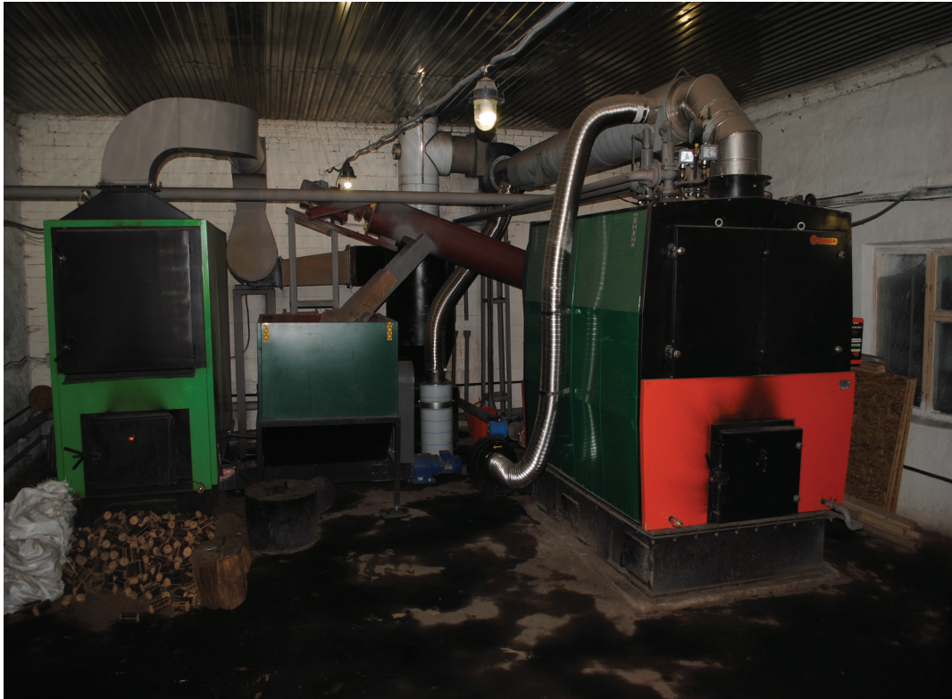
Fig. 6. Universal solid fuel boiler, VNAU
